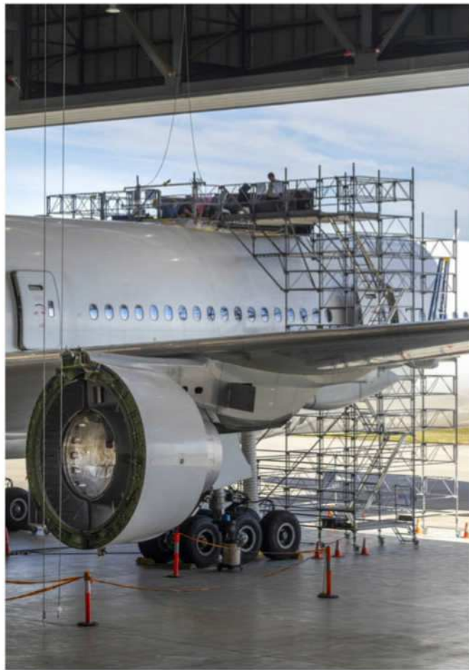
Installing the Wi-Fi radome on a Virgin Australia 777. SETH JAWORSKI
